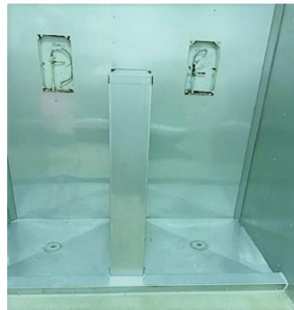
Shower stalls after refit
