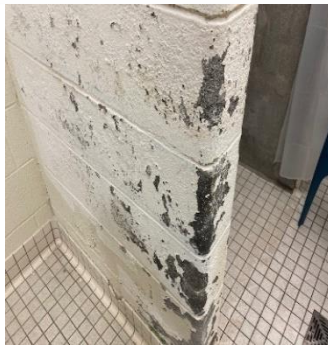
Shower stalls before refit
