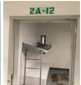
2AB upper bunk install
